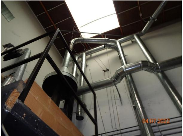
Details, Ø150 mm FFDT, mixing section, elbows and adjustable extraction hood
